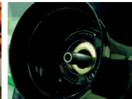
Aft drive adapter incorrectly installed. The propeller will fall off the propeller shaft if run with this incorrect installation.
